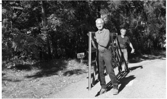
Gary Emanuel and Kenny Bales removing the old gate from the exit road.
