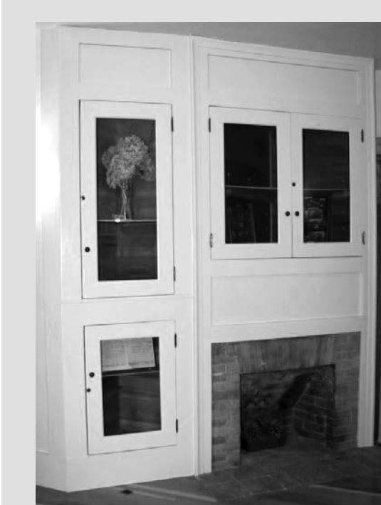
Volunteer Mark Glendenning made repairs to the Julia Morgan Room fireplace, and built and installed new cabinets containing artifacts donated by the Foote family descendants.
