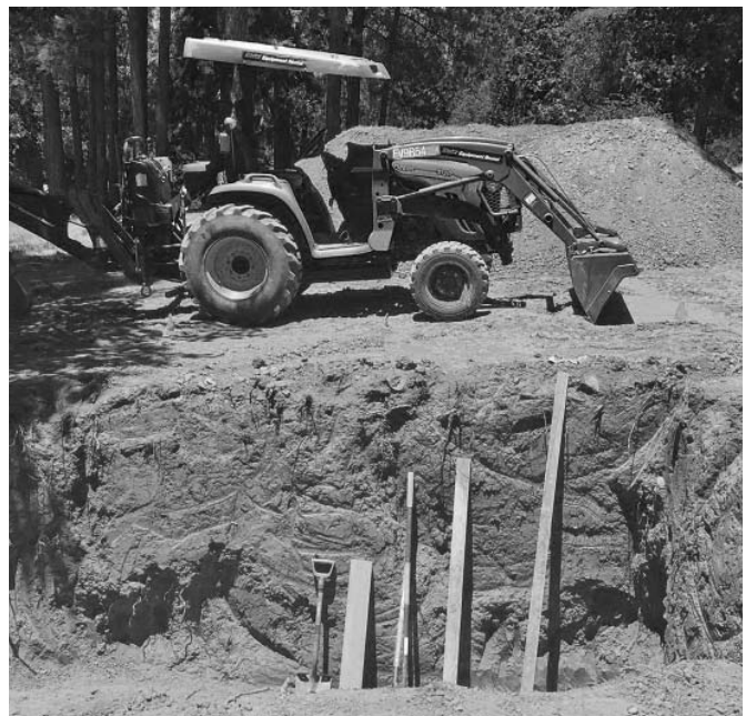
Excavation Complete; Bring on the Tanks!
