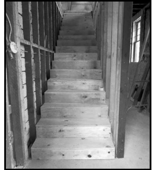
Staircase will serve as second floor emergency exit.
