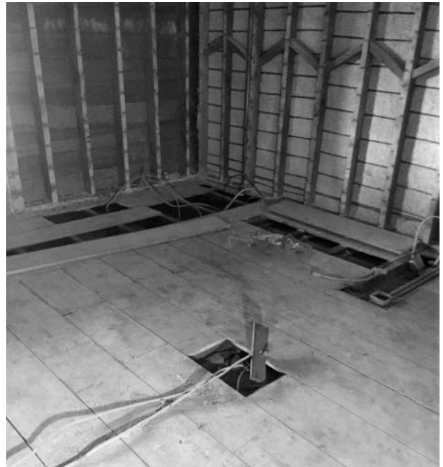
The future Art Gallery that is being used as access to the Living Room overhead lights. The flex cable will be removed after the new wiring is in place. Progress!
