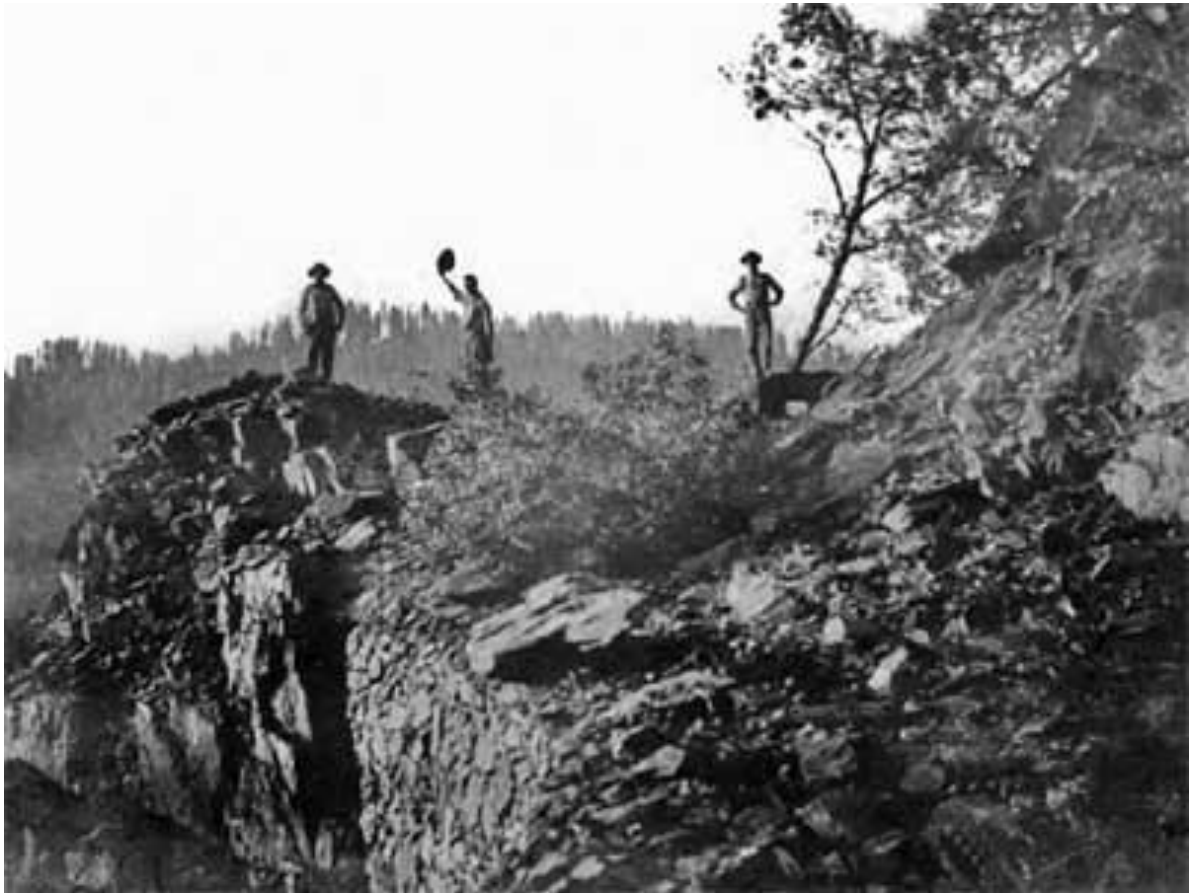
Foote's Crossing Road Workers, 1913
